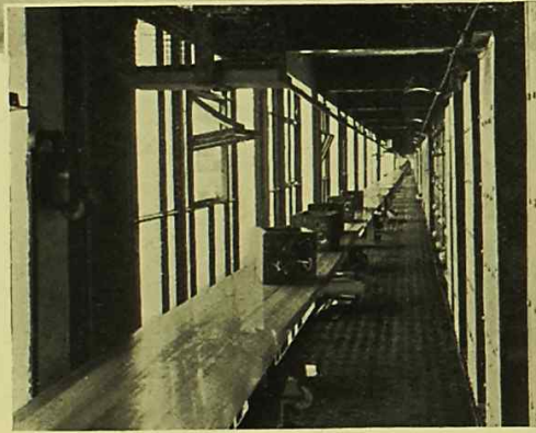
Above, Main Service Shop. Below, Parts Conveyor.
