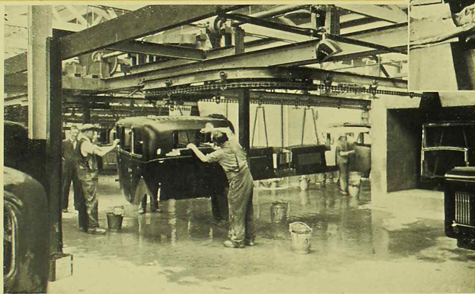
The continuous process painting plant — rubbing down.
